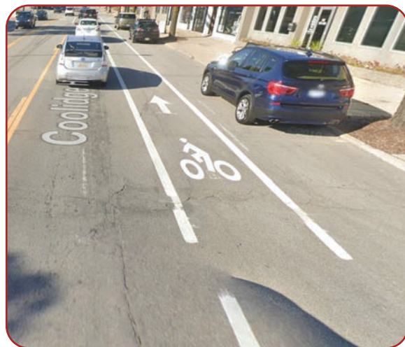
The road diet on Coolidge with on-street parking and a bicycle lane is an example of a Complete Streets improvement. Source: Google Streetview
