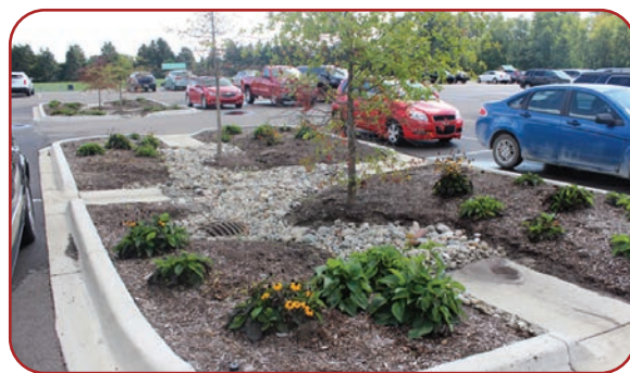
Green infrastructure in parking lot islands. Source: Presentation on Green Infrastructure Webinar
